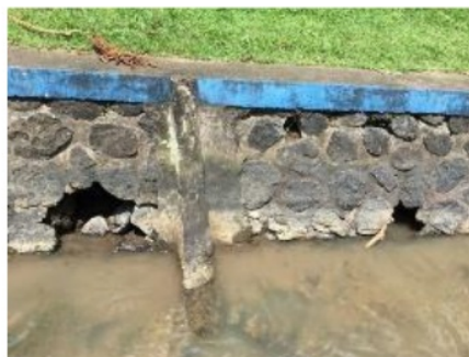
Picture 6. Channel Wall Damage Due to Erosion
