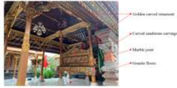
Figure 7. Implementation of Modern Materials, Colors, and Ornaments in Bale Delod Building Source: Author, 2021
