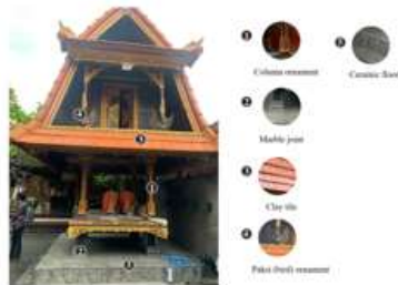
Figure 4. The Shape of The Jineng (Barn) Building which Has Undergone A Transformation in Form and Function Source: Author, 2021
