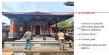
Figure 9. Implementation of Modern Materials in Bale Dauh Building Source: Author, 2021
