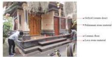
Figure 8. Implementation of Modern Materials and Ornaments in Kitchen ( Paon ) Building Source: Author, 2021
