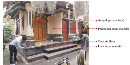
Figure 8. Implementation of Modern Materials and Ornaments in Kitchen ( Paon ) Building Source: Author, 2021
