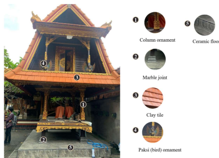
Figure 4. The Shape of The Jimeng (Barn) Building which Has Undergone A Transformation in Form and Function Source: Author, 2021
