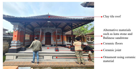
Figure 9. Implementation of Modern Materials in Bale Dauh Building Source: Author, 2021
