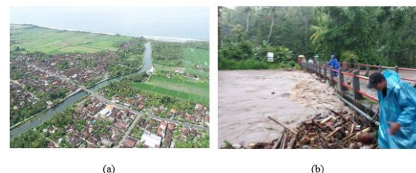
Figure 2. Yeh Embang Watershed in Normal Condition (a) and in Flood Condition (b)
