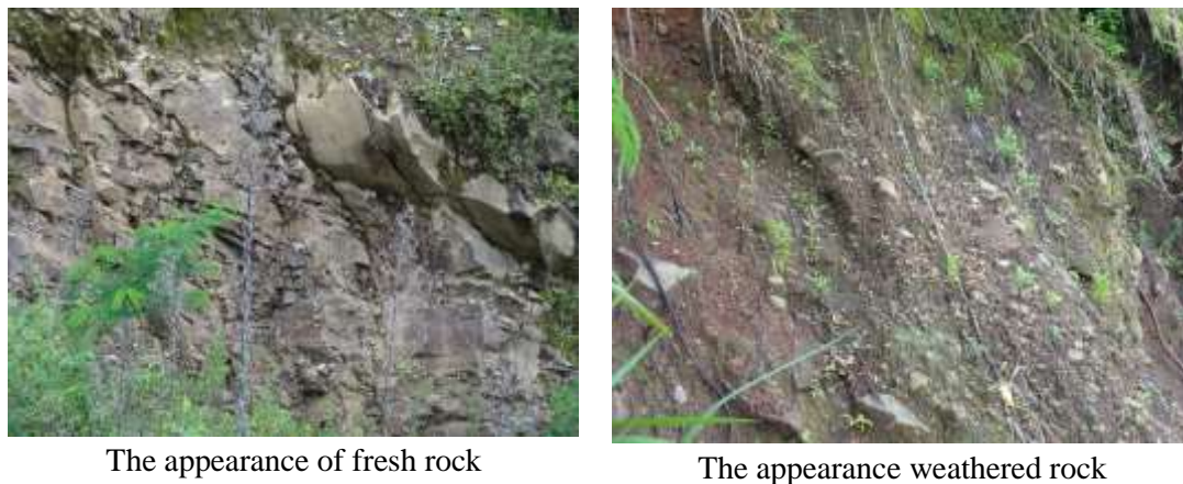
Figure 5. Slope outcrops in the study area
