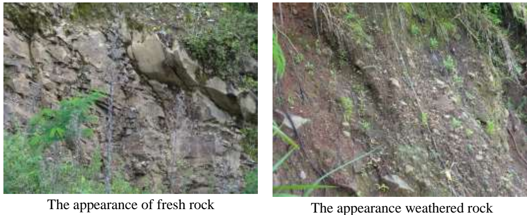
Figure 5. Slope outcrops in the study area
