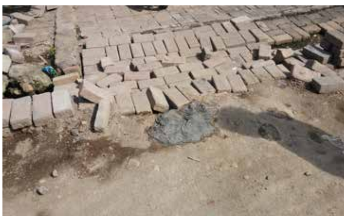
Photo 5. The covering street by using plastic disposal and the damage paving block in RT 05 RW 07 Kampong Kemijen (source: fieldwork on May 5 th , 2016).
