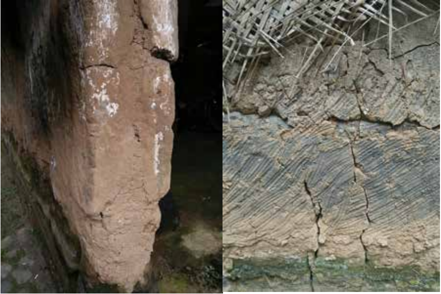
Pic 11. Wall of House with polpolan soil at Pondok Jaka Sangeh Source : Own doc, 2017
