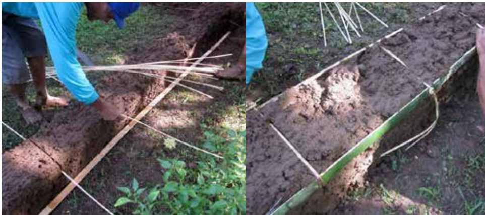
Pic. 7. Soil that begins to be arranged and clipped with bamboo frame Source: facebook green architecture, 2011
