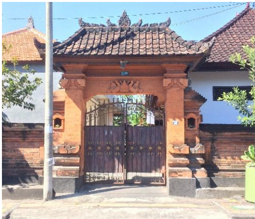
Figure 6. Angkul-angkul at Raya Pemogan Street No. 137 (Source: survey, 2017)
