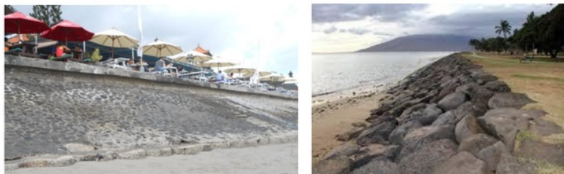
Figure 2. Revetment in General Source: www.google.com
